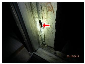
**7.1** (2) There is evidence of previous moisture staining on the walls/ceiling/floors of the air handler utility closet. These areas were tested and are non-resultant for active or elevated moisture levels.
