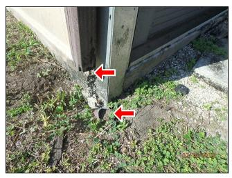
**2.3** (3) The gutters will need service in several areas, there are leaks at seams/end stops, water retention and debris in gutters/downspouts
