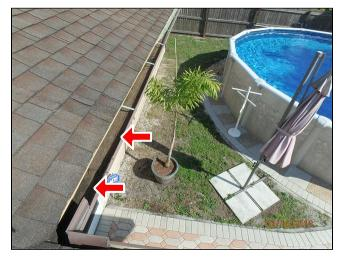
**2.3** (2) Physically damaged gutter downspout should be replaced and terminated further away from the structure to prevent eventual ground and soil erosion.
