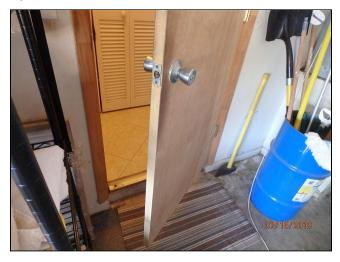
**10.5** Some wood rot/deterioration at the bottom of the lower portion of the door frame. This is typical for exterior doors subject to exposure to rain.
