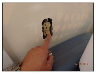
10.10 Open gaps in the garage walls should be sealed and finished to prevent moisture and pest entry
