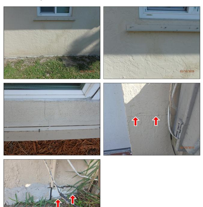
1.2 There is a soffit vent with wires going through it. The open gap should be properly sealed to prevent pest entry
