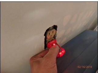
10.9 Loose receptacle and missing a cover plate
