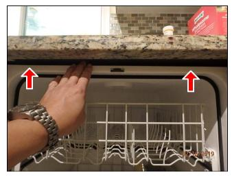
**3.0** (3) The dishwasher operated as expected. However, there is no high loop or air gap installed at the dishwasher. A high loop or air gap functions to not allow (dirty) water to back into the appliance and acts as an air gap and trap to prevent back flow of gases. Recommend proper installation even if the appliance has one built in on the inside.
