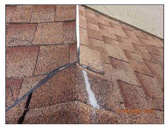
**2.1** (2) There are one or more areas where flashing/kick out flashing is missing or may be inadequate to effectively divert water away from the house. Missing, inadequate or damaged flashing can cause leaks and water intrusion into the home.
