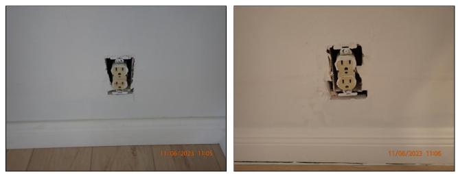
**6.5** (1) Loose receptacle(s) should be properly secured to prevent movement
