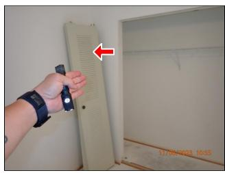
**4.3** There is visible mold present. There is also musty odors which are indicative of the presence of active mold. We recommend having a mold assessment conducted in order to confirm the presence of mold, the type of mold and mold spore counts to ascertain the level of danger in the structure. All visible mold and the sources of moisture will require remediation.
