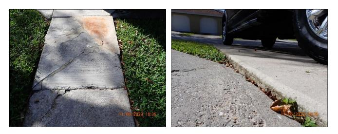
**1.5** (2) Walkways are sinking and causing a trip hazard. There is a large tree nearby and the root system can be affecting the walkways and drvieway. This needs to be corrected as it is a tripping safety hazard.
