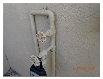
**7.0** (2) The main water shut off is a gate valve design. These are not tested as part of the inspection due to potential failure. It is recommended that at your convenience this valve be replaced with a quarter turn ball valve design
