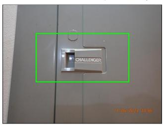
**6.2** (2) Improper distribution panel screws. Correct screws have a flat tip so they would not accidently penetrate a wire inside the panel. Recommend replacing any improper screws with the correct panel screw types.
