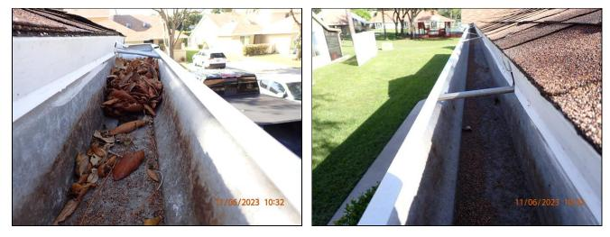
**2.3** (2) There are seams in the gutter system that appear to be leaking. These seams should be properly sealed.
