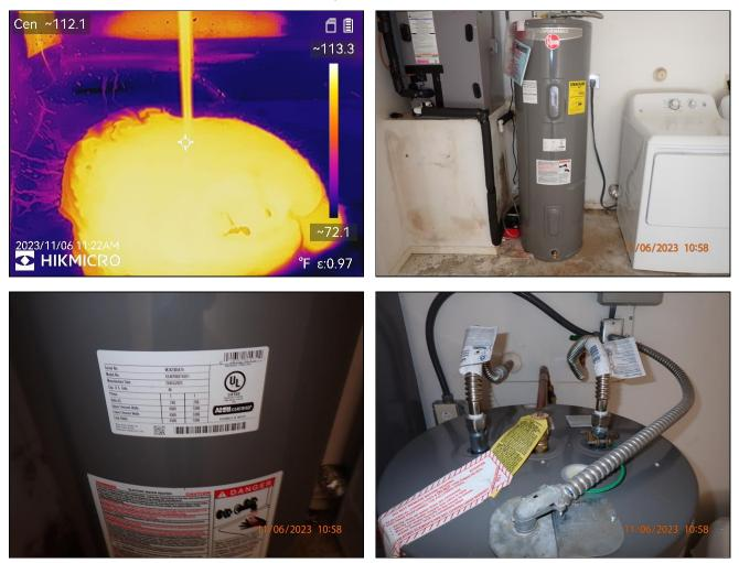
7.4 (2) Water heater was inspected and scanned with a thermal camera and was not leaking at the time of the inspection.
