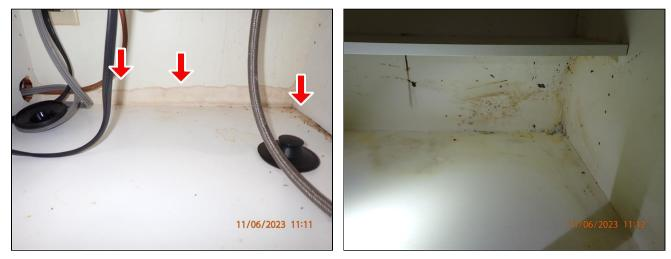
**4.1** (2) Kitchen sink cabinet has damages to the floorboards and walls.
