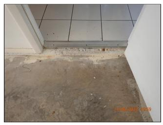
**3.3** (2) The occupant door from the garage to the interior of the house should seal properly to prevent odors and fumes from entering the home. An improper or inadequate seal can allow poisonous CO gases to enter into the home under certain circumstances. Recommend checking the seal periodically to ensure it is intact and making a proper seal and replace as necessary.
