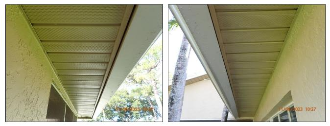
**1.1** (2) There are one or more areas along the fascia that appear to have some degree of moisture deterioration. Recommend monitoring this area and replace if necessary. Presence of moisture or prolonged presence of moisture would indicate possible roof leaks in the affected areas. Note: When opening these affected areas up for repair/replacement, expect that there will be some degree of deterioration with the fascia, sheathing and or other concealed components.
