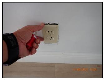
**6.5** (2) One or more receptacles are painted or otherwise has openings restricted and the tester could not be inserted in order to test the outlet. The functionality of the outlet is not known. The polarity and grounding of that outlet is not known.
