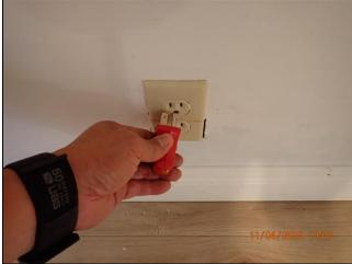
**6.5** (3) One or more interior receptacle did not have power. The electrical system will require further evaluation and correction.
