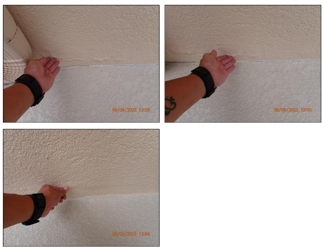
**1.1** The visible eaves, soffits and fascia all appear to be in good overall condition. There are no visible water intrusion damage or wood rot or deterioration noted. Note that a visual inspection from the ground is limited and concealed damages and deterioration behind painted surfaces are not usually visible. There are at least two areas of water leaking which can be seen from inside the attic.
