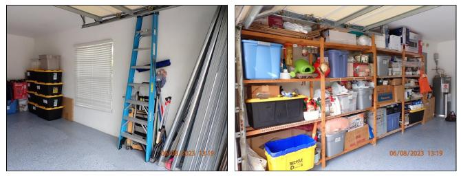
**3.1** The garage floor has been covered with an epoxy type garage floor paint system. The concrete underneath is not accessible. Looks to be in good overall condition.
