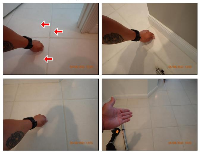
4.2 Closet door binds at a certain point because the roller system is making contact with a part of the flooring.
