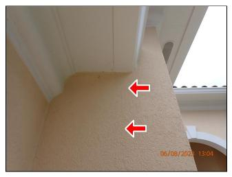
**1.0** (2) There are a few areas of the finished exterior surfaces where moisture is likely causing some degradation of the stucco.
