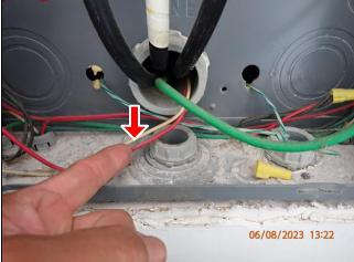
**6.2** (2) Wrong type of screw being used at the service disconnect.
