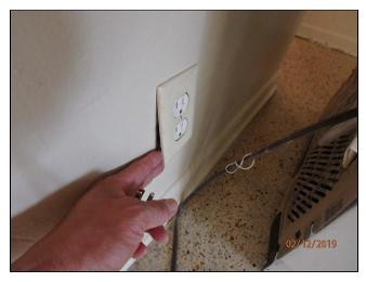
**5.5** (2) Improperly/inadequately grounded receptacle. Should be corrected by a qualified electrical contractor
