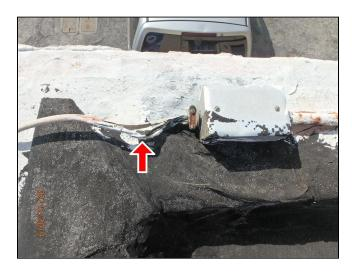
1.12 Open gaps in exterior walls should be sealed and finished to prevent moisture and pest entry.
