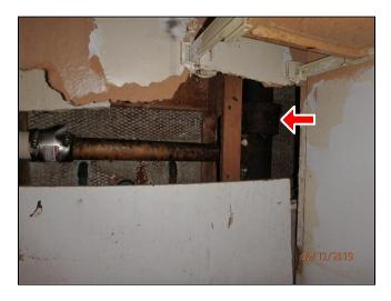
**6.1** (2) There is aged cast iron piping at the rear of the exterior of the front building. It is unknown whether or not it is still being used. But it is not properly secured to the wall and it has detached piping. This pipe should be corrected and secured or removed and capped off.
