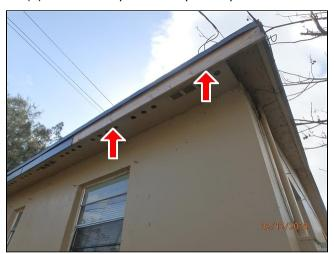
1.2 (2) Areas of deteriorated soffit trim
