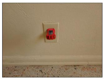
**5.7** There are some receptacles in the bathroom/kitchen(s) within the proximity of a sink/vanity which is not GCI protected. It is recommended that these receptacles are replaced or are protected up stream with a GFCI protected receptacle.
