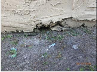
1.13 The exterior water heater shed is deteriorated and has termite damage to the framing
