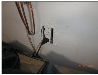
5.5 (1) Loose receptacle(s) should be properly secured to prevent movement
