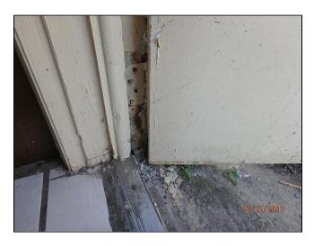
1.4 Window not properly sealed will allow moisture and rainwater to penetrate and cause moisture damage
